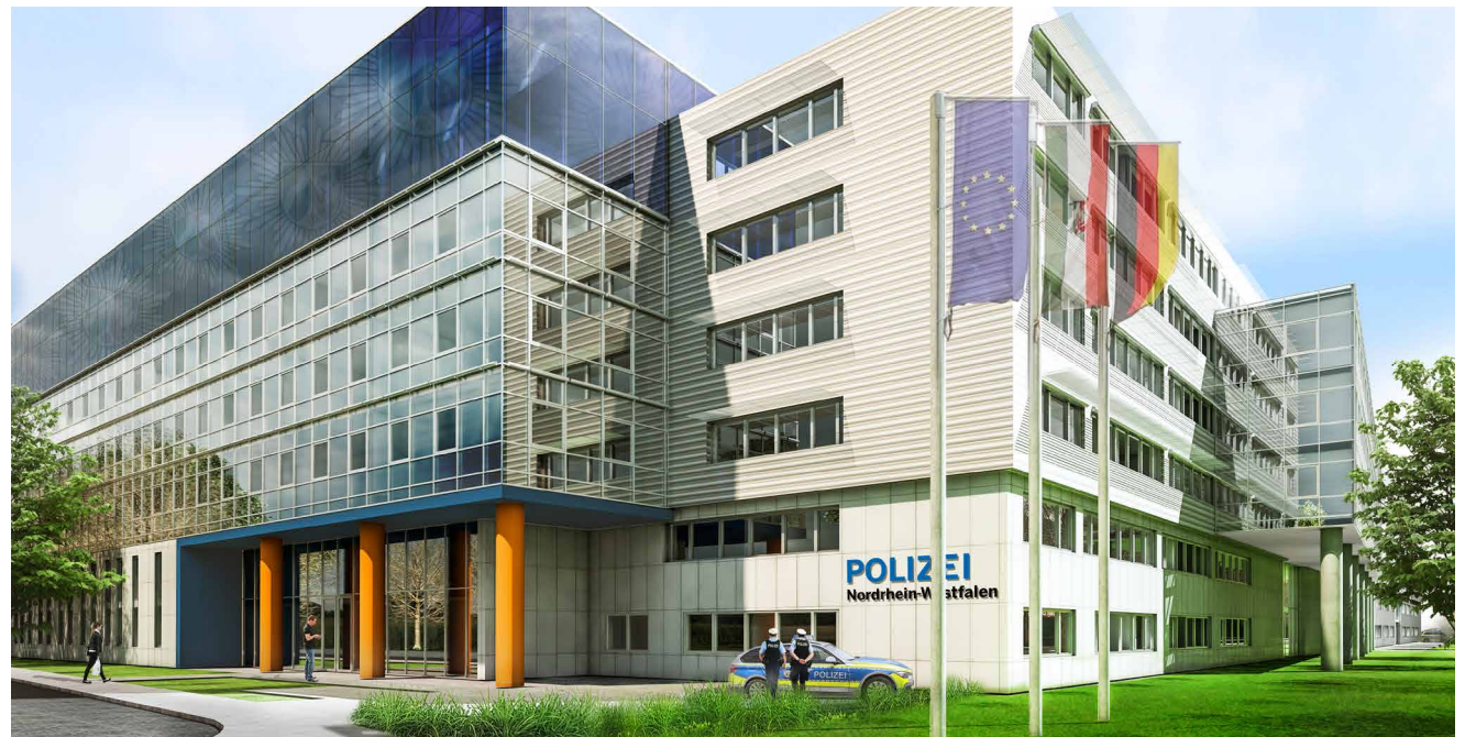
Essen Office Park Bredeneu: The lease agreement was concluded for 20 years; occupation by the Essen police is planned for 2025.
